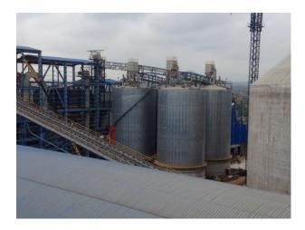
This "satellite" grinding plant will receive clinker and additives from thru the nearby port. To do so, a material receiving system with a 50'000 T clinker silo and an additive storage facility for gypsum, limestone, BFS and a separate storage silo for fly ash is available.
